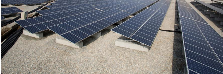
**ON THE GROUNDS OF JAPANESE RADIO** and TV station BSS (Broadcasting System of San-in) in Yonago, more than 7,000 REC solar panels are installed – creating a 1.7 MW power plant that produces enough electricity to power 510 Japanese households.
