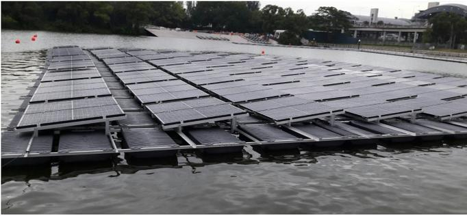
Constant movement of the floating platform on the water adds mechanical stress - firstly to the underconstruction with a potential secondary effect on the solar panels and cabling system. This is dependent on pontoon design and how rigid or flexible the mounting structure is. Movement of the pontoon also stresses the mooring system, so this also needs regular checks to ensure optimum safety.
